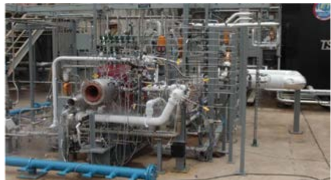
Figure 4: Test Stand 116 pump-fed position (AMDE setup).
