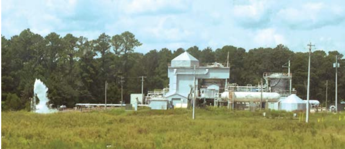
MSFC's Test Stand 300 during liquid nitrogen testing—Phase A of IVF.
