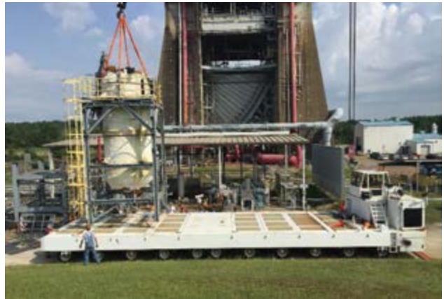
Figure 2: Relocating 10,000-gallon tank to TS 116.
